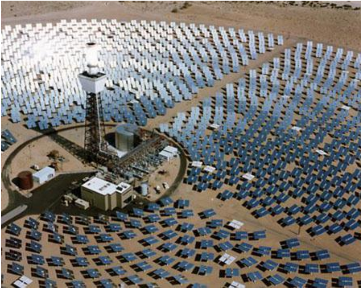
Power tower in Barstow, California.
