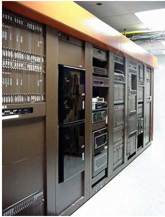
Telecom Systems And Networks
