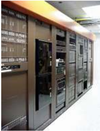
Telecom Systems And Networks
